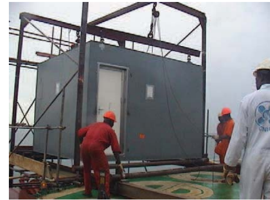
Modules installation on board
